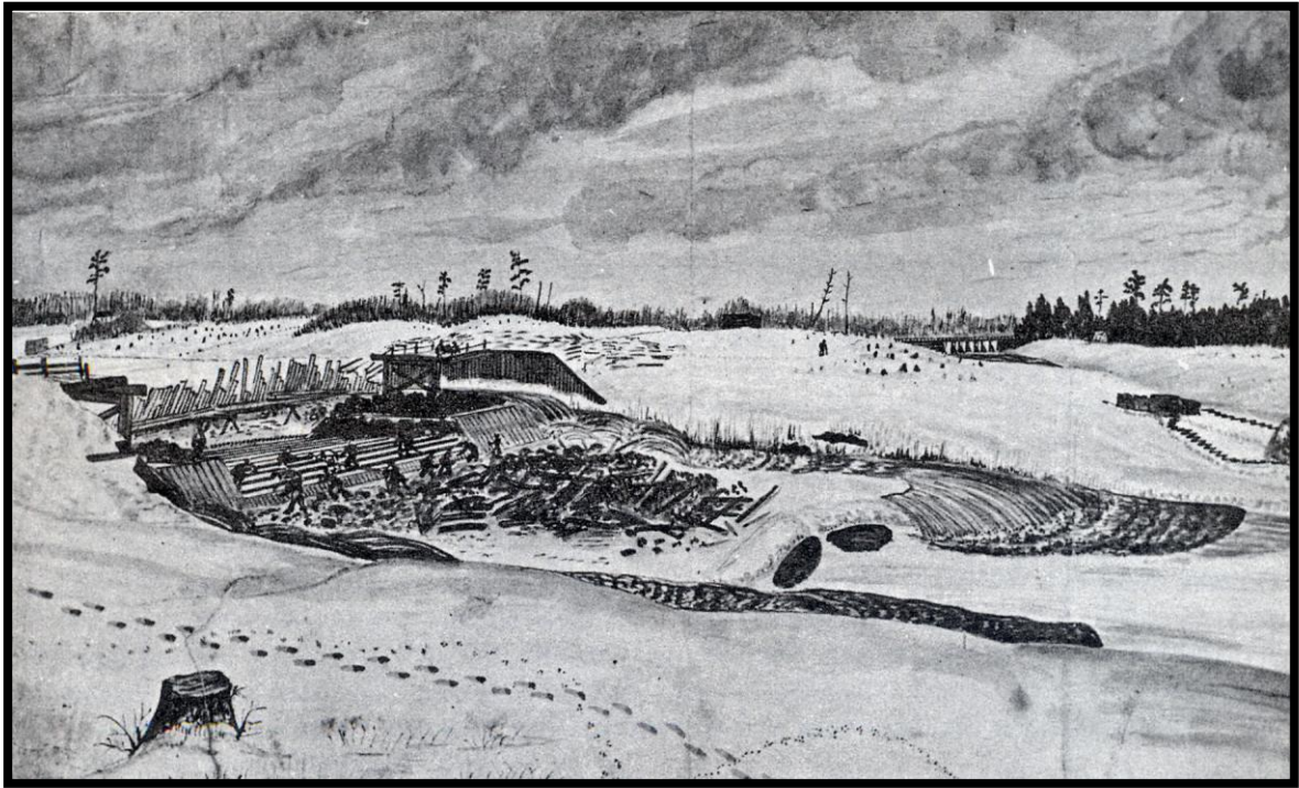
Figure 15. Repairing the waste weir dam at Long Island in February 1845 - the Mud Creek waste weir is in the right background. Sketched by Thomas Burrowes. (Ontario Archives.)
